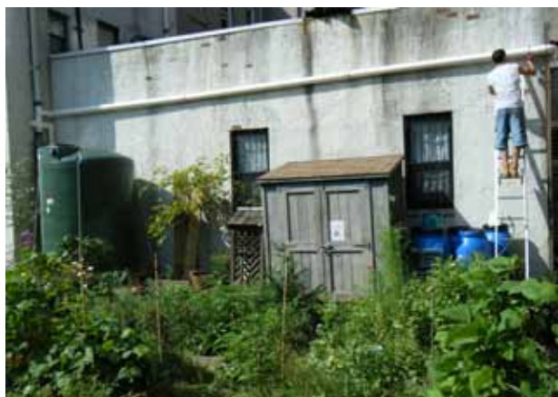
Installing a roof collection RWH system
